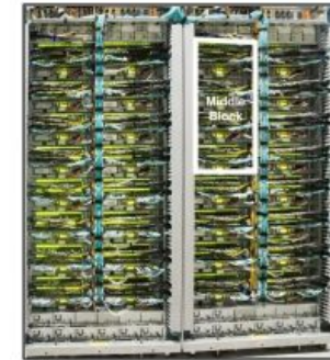
Figure 14: Jupiter Middle blocks housed in racks.
