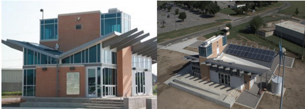
Figure 1: Zero Energy Building, where the experiments took place.
