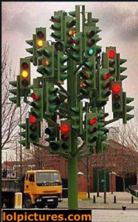
Traffic Light Controller
