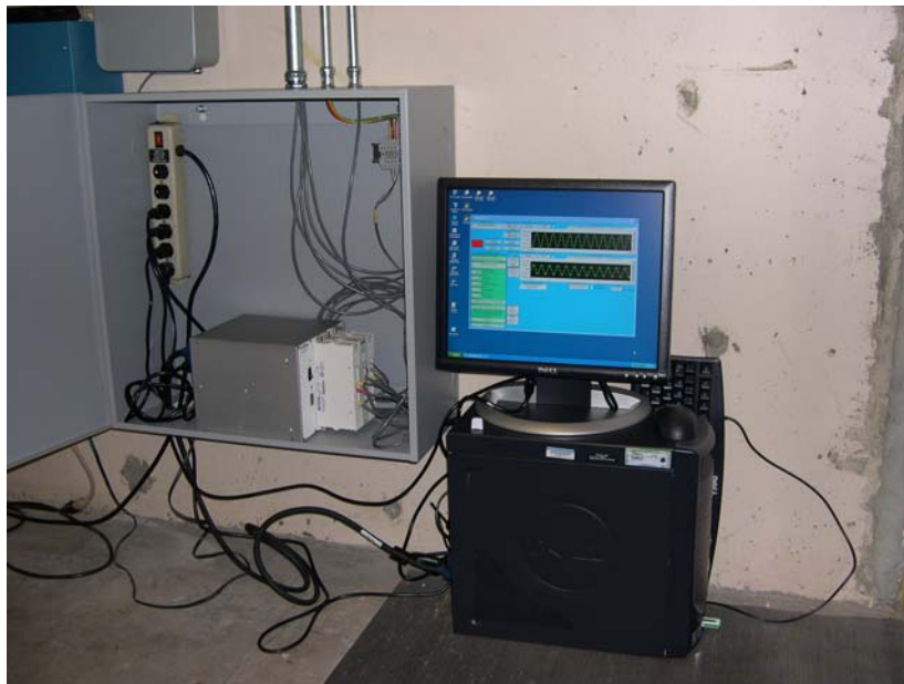
Figure 9 PPSM Monitoring Unit at BPA's Portland Headquarters
