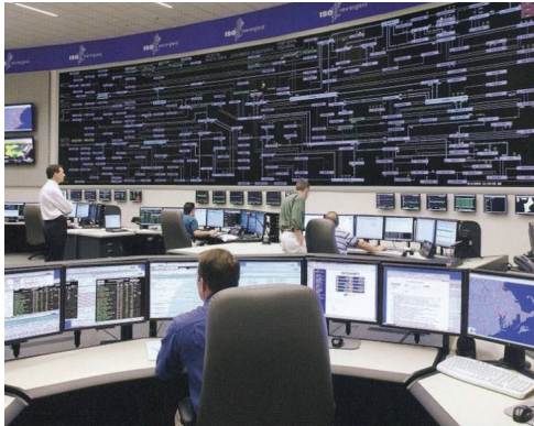
Control room of a transmission system operator
